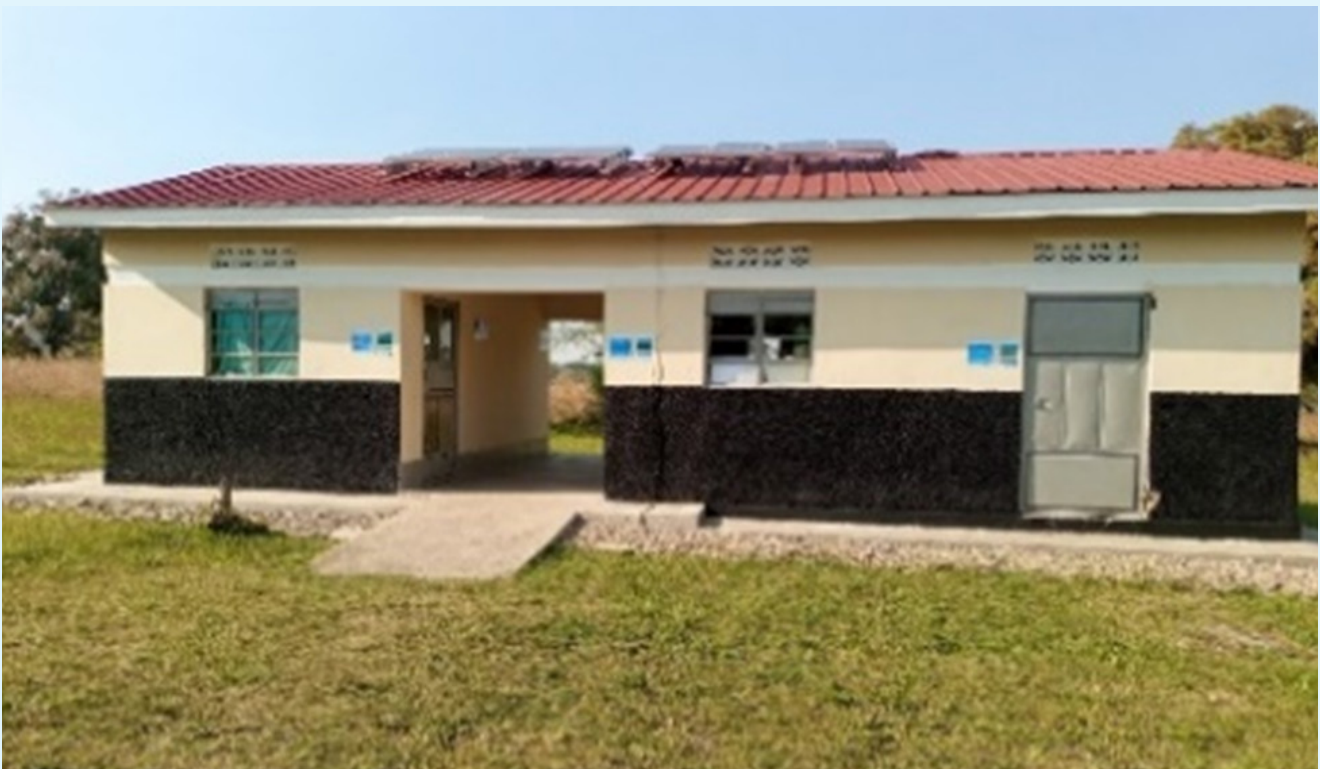
▲ Mere PHCU building after the renovation
